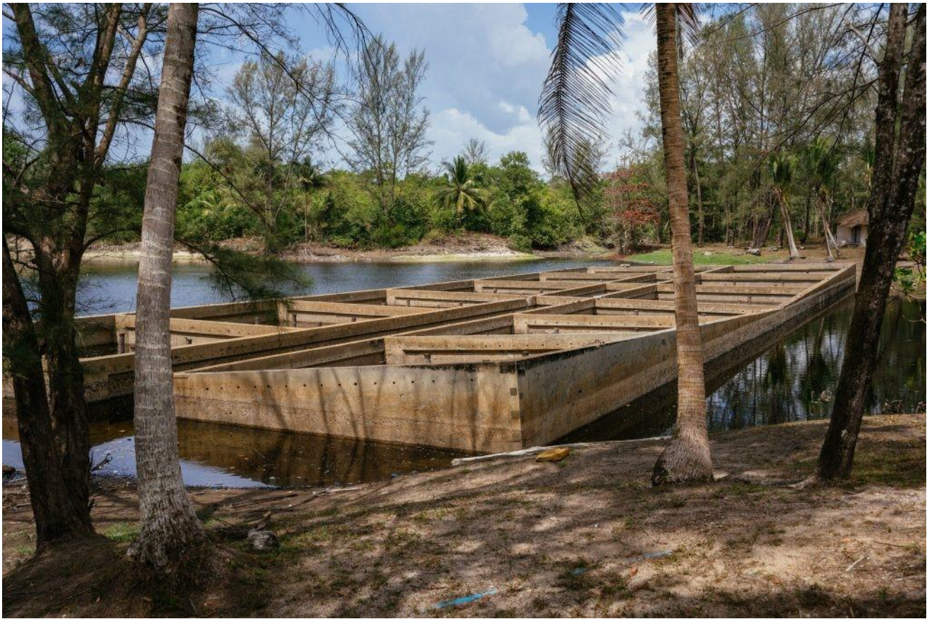
Within this national park, there are also the remains of Thailand's first dredger, a large mining dredger located in a water reservoir within the pine forest along the beach. The structure consists of large concrete sections divided into compartments and was built between 1975 and 1977. It was designed as a floating dredger in a dock dug along the beach to create space for mining activities. However, before the dredger was completed, the concession owner canceled the mining project, leaving only its remains visible today.
